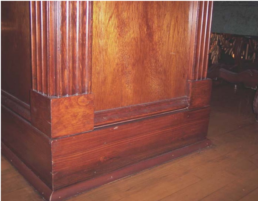
PRE-STAINED BASE SHOE AWAITING FURTHER WORK
