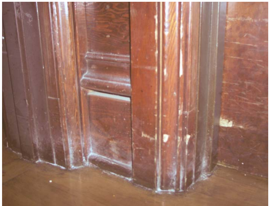
CLEANING PRODUCT BUILDUP AND CHIPPED WOOD
